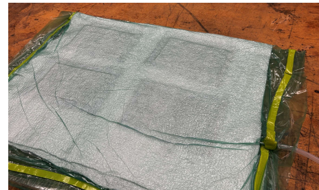
Figure 37. Vacuum Bagging Setup
